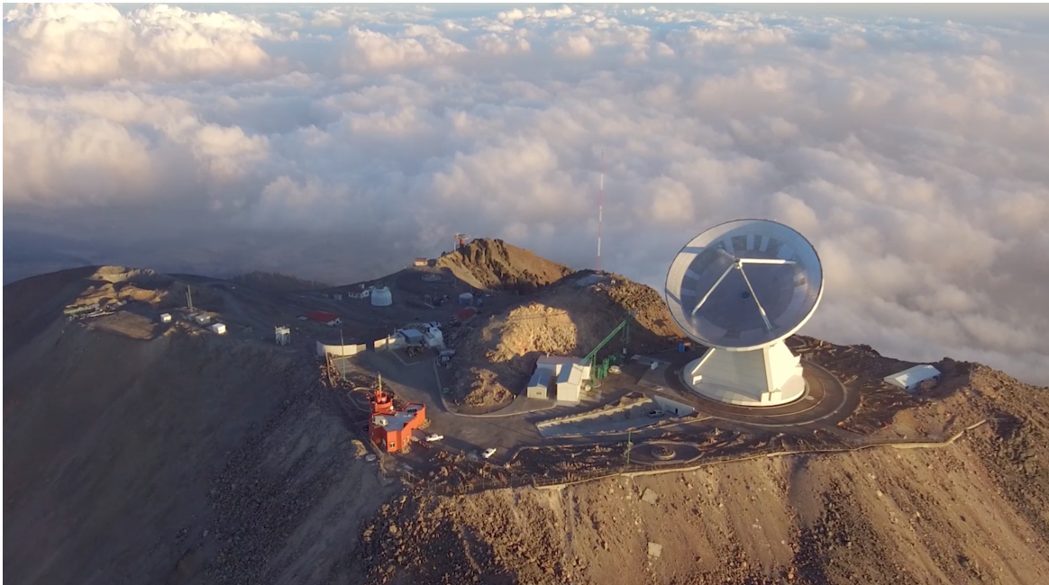
Figure 2. Aerial view (late afternoon) of the summit of Volcán Sierra Negra (altitude 4600m). The site shows the LMT pointing north. The electrical substation, workshop and metrology building can be seen to the left of the telescope, and above the ramp. The green tower-crane (in its lowered position) provides access for installation and maintenance to the secondary mirror, hexapod and segments of the primary reflector (M1), as well as providing the platform to conduct photogrammetry measurements of M1. The red building is occasionally used as a visitor center, and the meteorological equipment including the 225GHz radiometer and external cameras are installed on the roof area of this building. Multiple lightning protection towers are distributed around the summit site.
